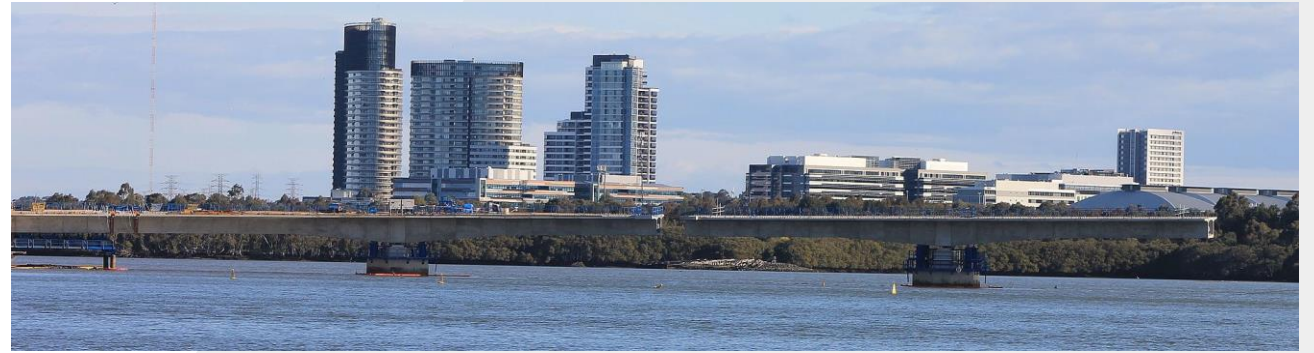
The bridge under construction
