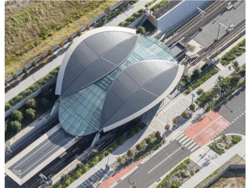
Bella Vista Station
